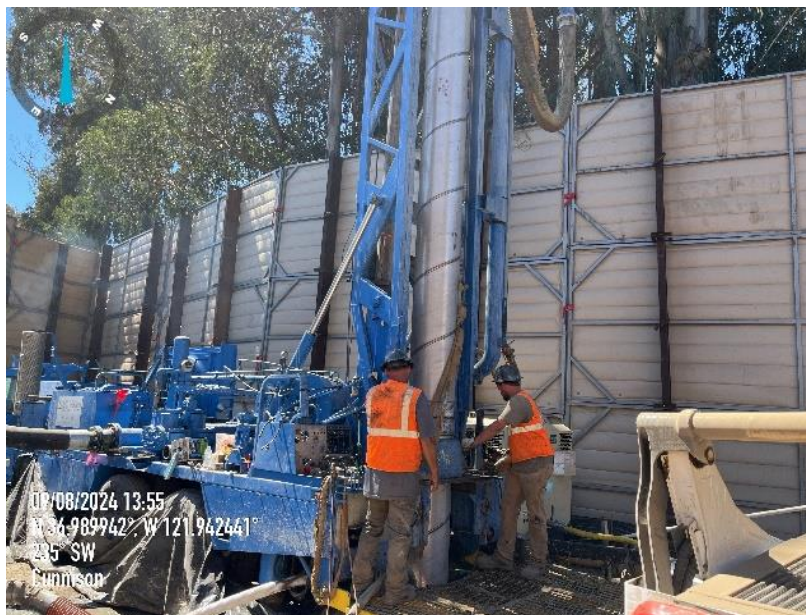
Figure 6: Cunnison Well drilling. Photo courtesy of SqCWD.
